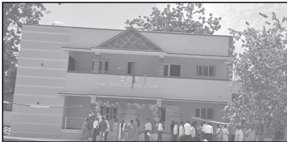
The New IBT Children's home building built in Bappanpalli, Odisha.
